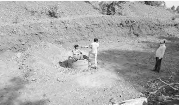
Artificial recharge pit in river bed rock
